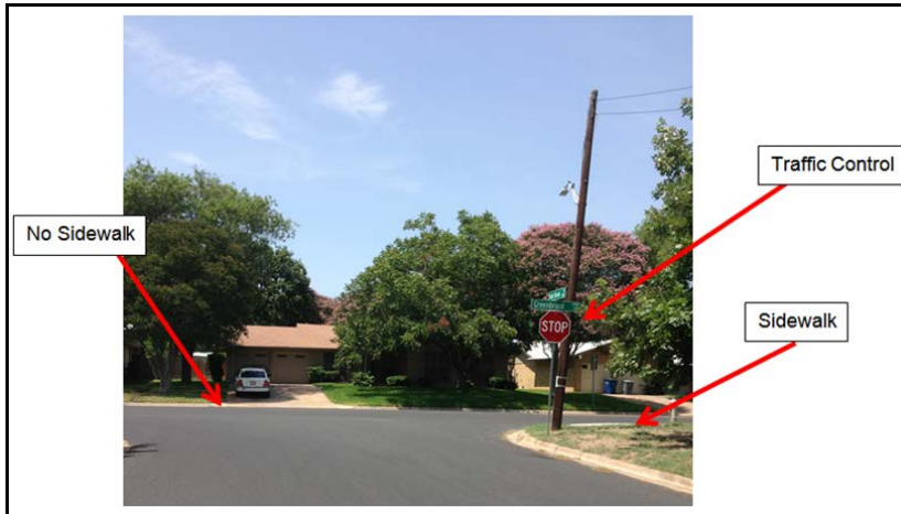
Figure 4: Caption: Photo of a t-intersection: The northbound street t's into the east/west street. A stop is on the northbound street (traffic control). The east/west street has no sidewalk on the north side. It does have sidewalks on the south side. The northbound street has no sidewalks.
