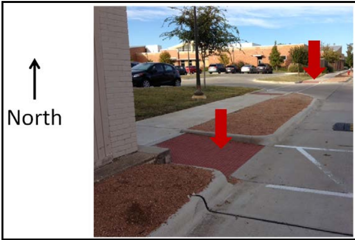
Figure 15: Photo shows two red arrows indicating ramps at sidewalks stop points.
